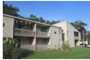
Multi-Family Property Jacksonville, FL
