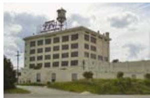
Industrial Property Richmond, VA
